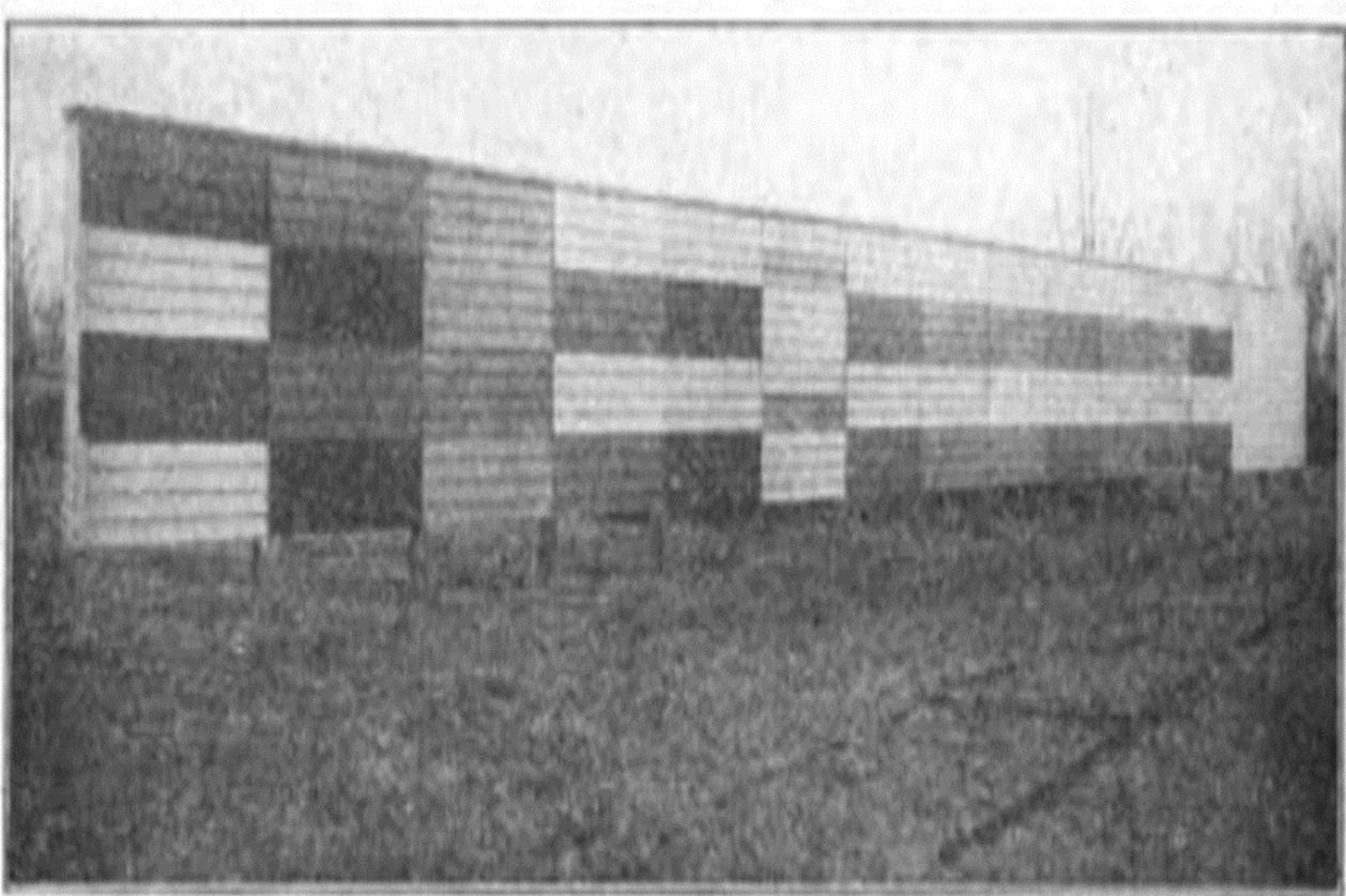
**Figure 1:** Earliest reported paint weathering “test fence,” 1906, Fargo, ND, faced east and west. Rusting nails stained the coatings.
